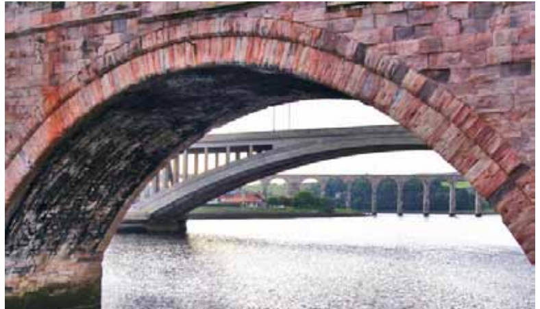
The old bridge, new bridge and viaduct Malcolm Morris, Geograph (Creative Commons License)
